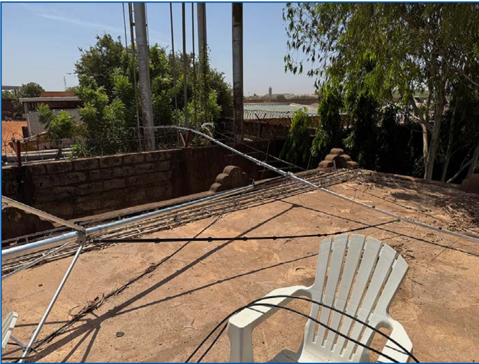
After some strong winds, I found the EME antenna lying on the roof, entangled in barbed wire.
